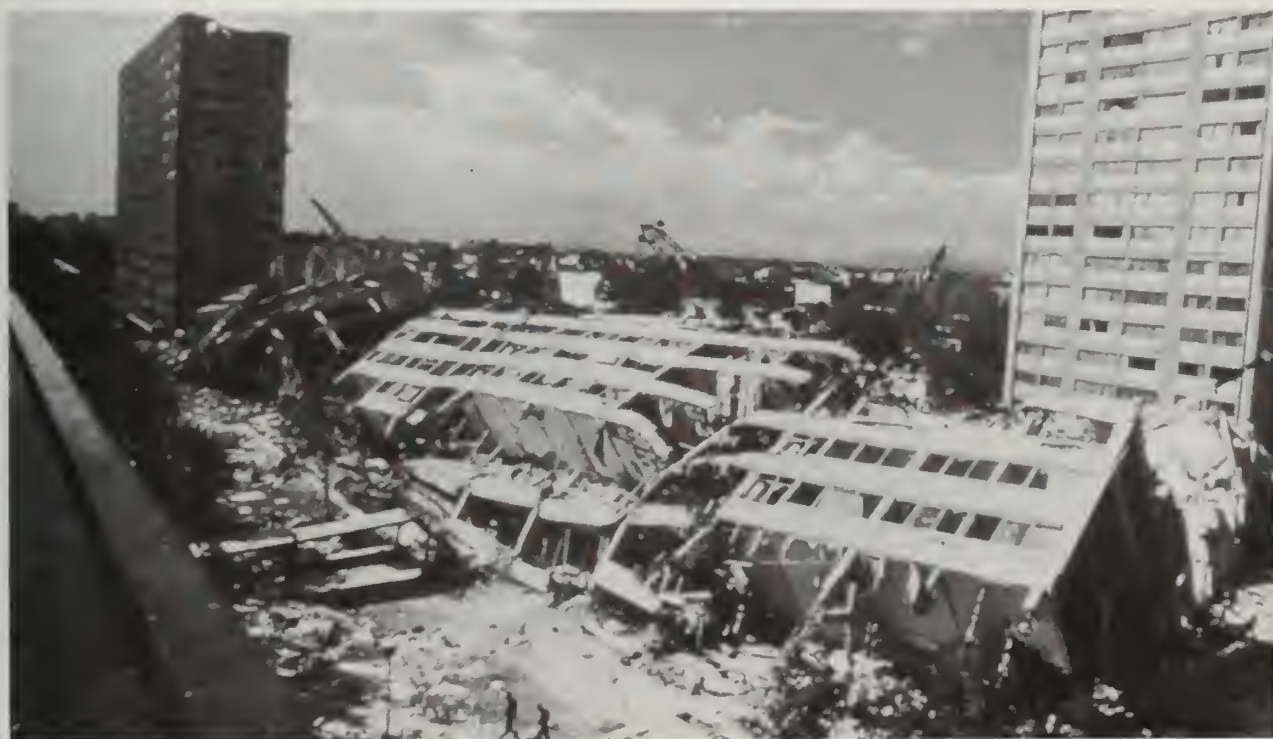
Collapse of the Nueva Leon apartment buildings caused by the 1985 Mexico City earthquake. The soft lake bed deposits amplified ground motions to damaging levels at distances exceeding 200 miles from the epicenter. Photo from Earthquake Engineering Research Institute.
